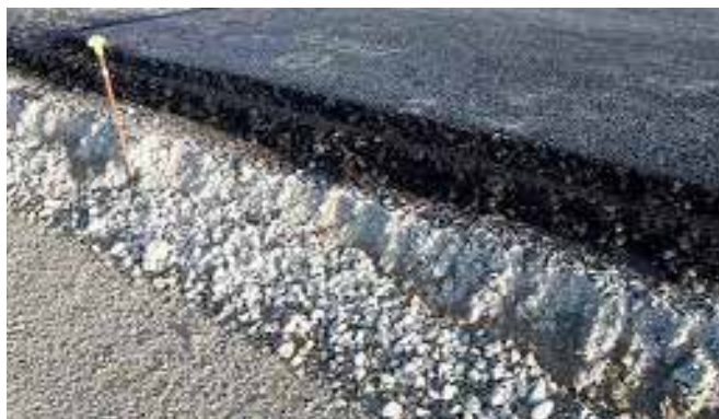
Figure 1: Typical asphalt placement and completed layers
